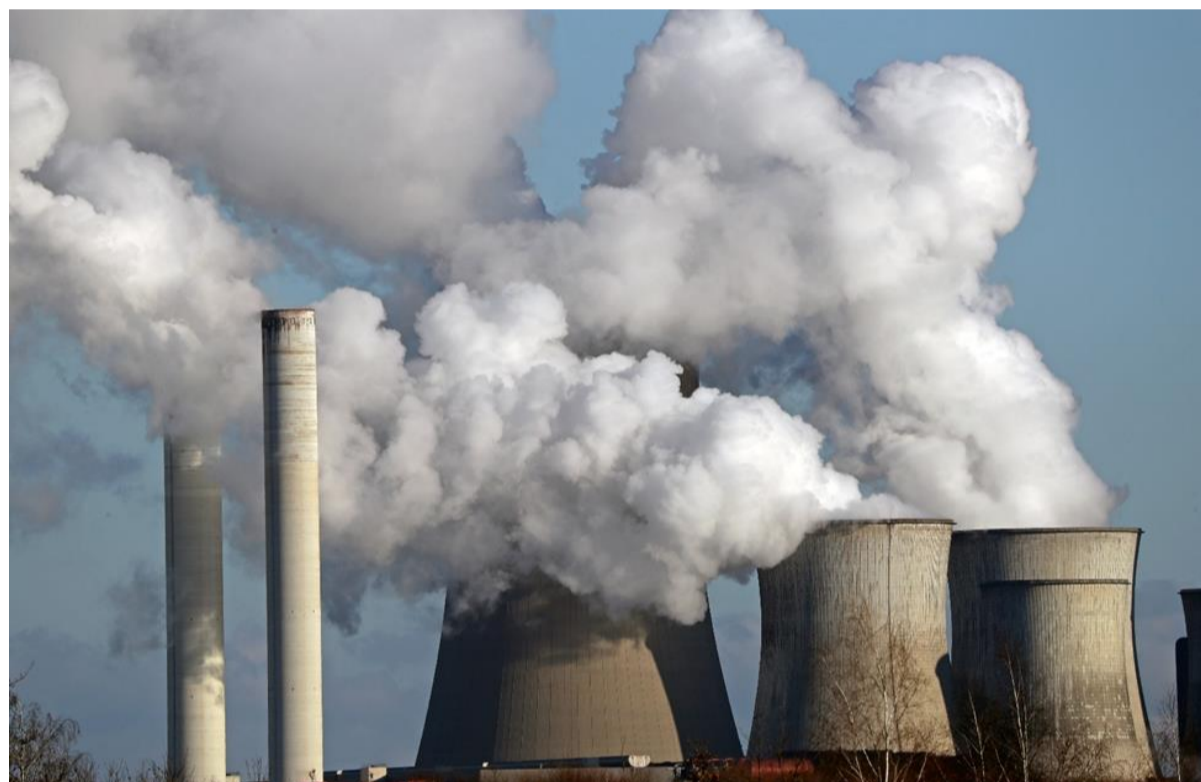
Niederaussem lignite power plant, in Niederaussem, Germany
